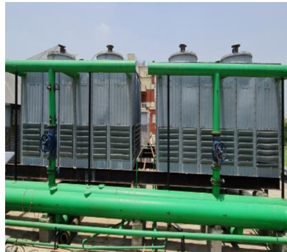
Cooling Tower Upgradation
