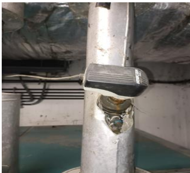
Actuator valve replacement
