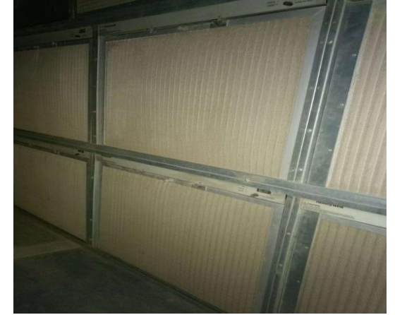
ESP Filter Retrofitting
