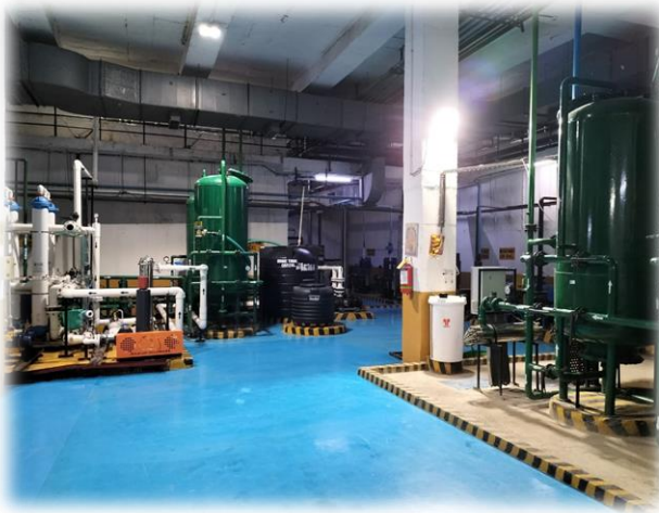
SEWAGE TREATMENT PLANT
